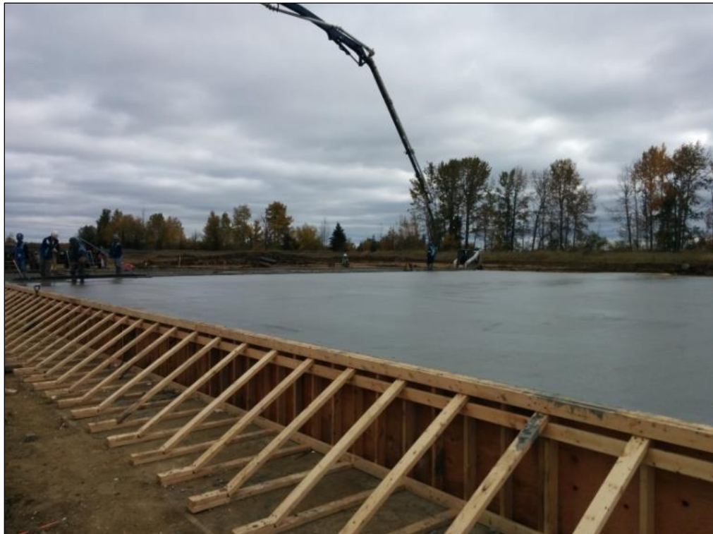
Photograph No. 2: Photograph showing the completed pour of the 700 m 3 slab.
