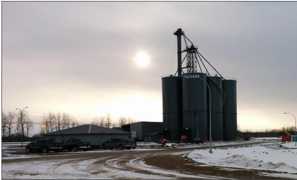
**Photograph No. 3:** Photograph showing the completed construction of the silos on the 700 m<sup>3</sup> slab.
