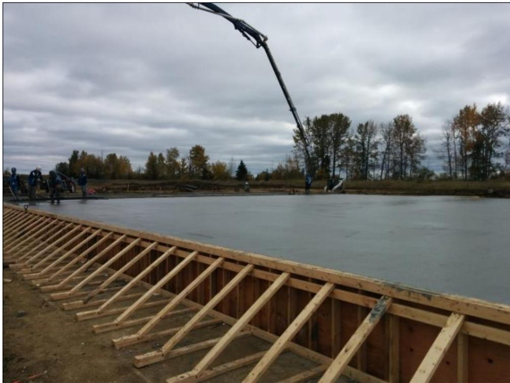
**Photograph No. 2:** Photograph showing the completed pour of the 700 m<sup>3</sup> slab.
